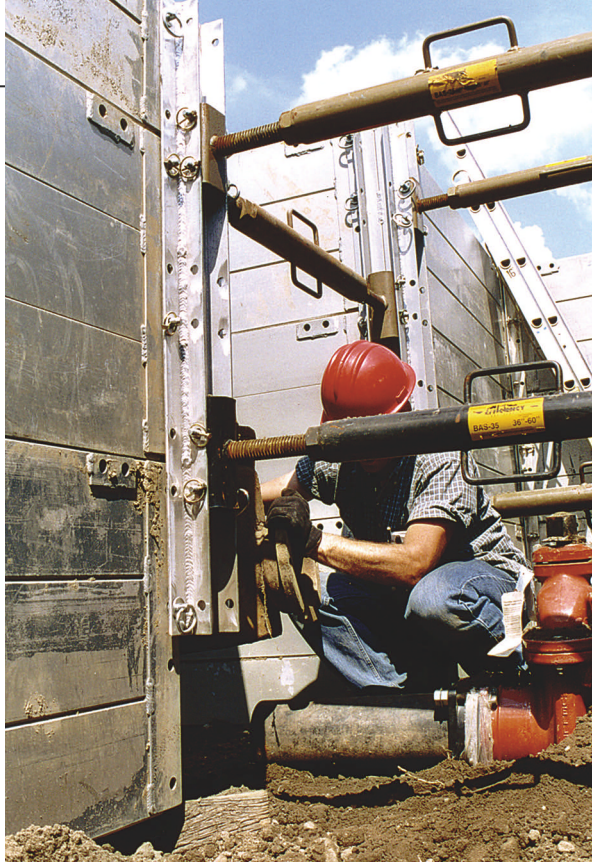
Trench safety must never be overlooked or disregarded. Shoring or trench boxes must be used to protect workers from collapsing sides.
