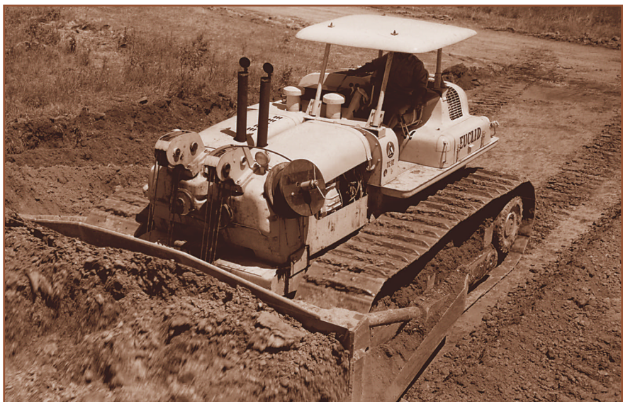
The first production TC-12 crawler tractors, designed and built by General Motors, were rated at 402 net horsepower.
